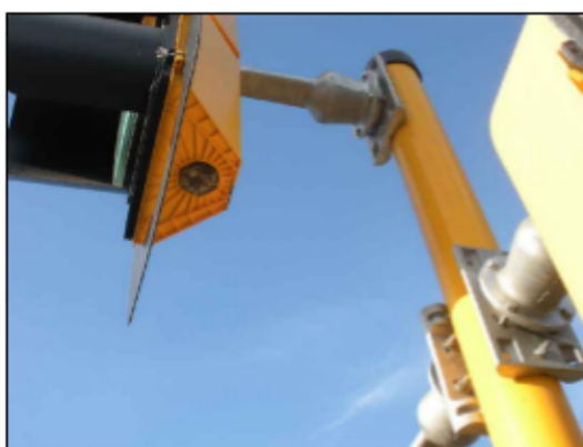
THRU-BOLT ADAPTER FOR POLE OR MAST ARM
