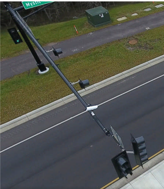
Strap-on style 5' Mast Arm Extension with Two-way signal mount.
