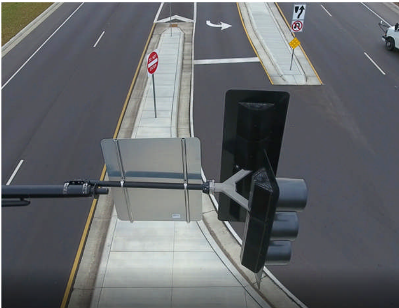
Strap-on style 5' Mast Arm Extension with Two-way signal mount.
