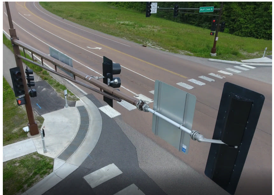
Clamp-on style 5' Mast Arm Extension with Angle signal mount.
